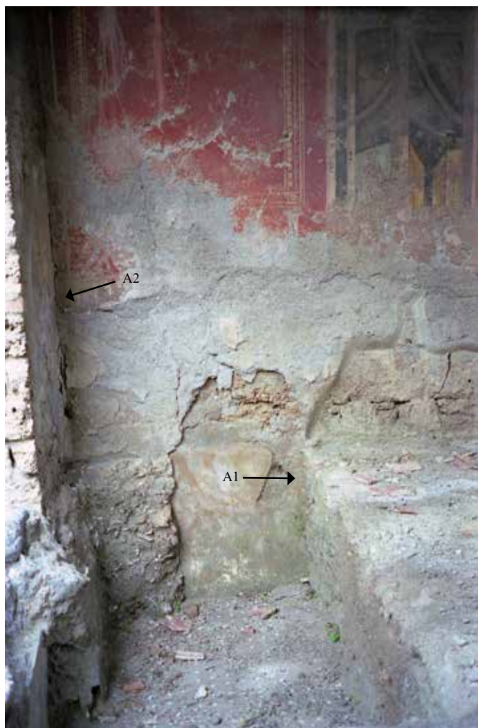
Fig. 2. Casa di Amarantus. Relative chronology of plaster layers in room 5, tablinum . The yellow socle is part of the original First Style decoration. The floor level was raised in the 1st century AD and the room redecorated in the Fourth Style.
