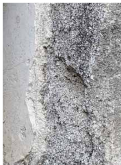
Fig. 3. Temple of Jupiter. A fragment of First Style plaster and white stucco on the west podium wall is trapped behind the abutting arch. Two layers of plaster and two of stucco are discernible. Also note the smooth stucco surface.
